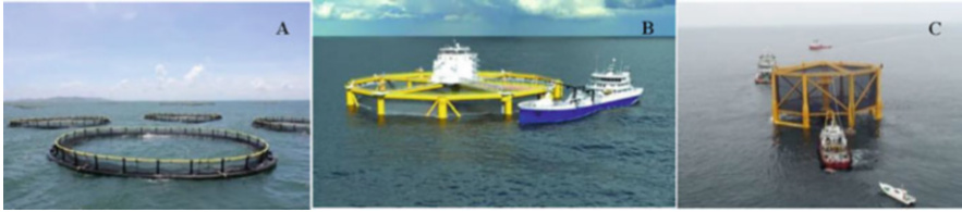
Fig. 12.1 Floating (a), semi-submersible (b), and submersible (c) aquaculture cages (Photo B from the internet)
