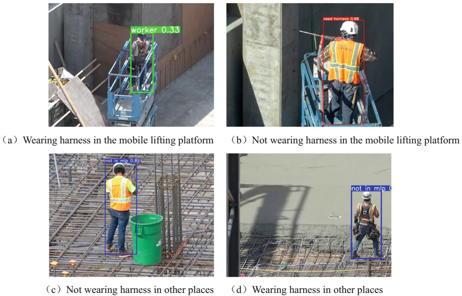
Fig. 4. Examples of the harness wearing condition detection output
