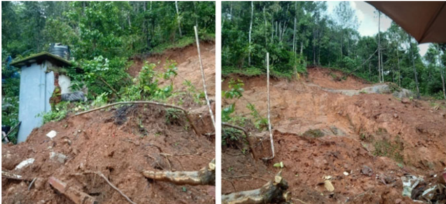
Fig. 6 House completely destroyed by a minor landslide on August 7, 2019
