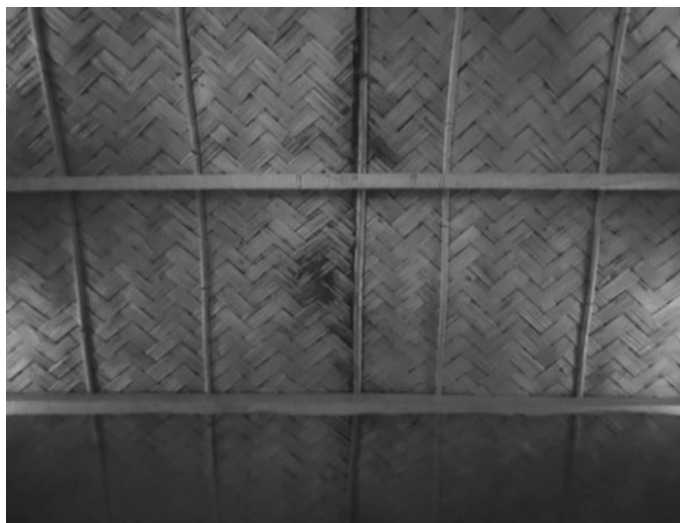
Fig. 8 Ceiling of the house
