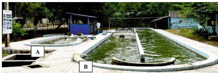
Fig. 4 Open raceway pond—capacity. (a) 5000 L and (b) 35,000 L
