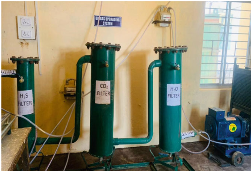
Fig. 1 Pressure swing adsorption-based filter unit
