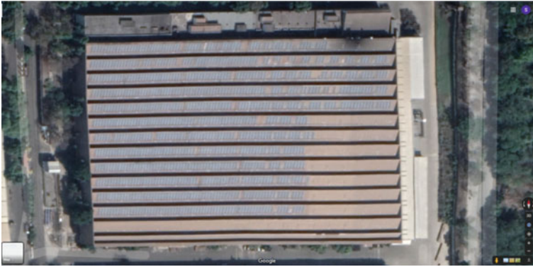
Fig. 3 Actual site photographs of 1.43 MWp rooftop solar PV plant
