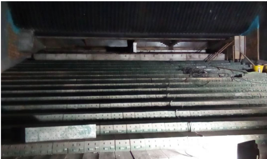
Fig. 7 Reciprocating grate inspection after six months operations
