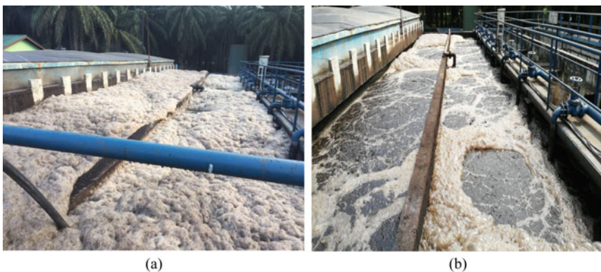
Fig. 10 Day 1: 30 March 2018 (a) 5 April 2018 (b) Foam condition after 5 days with Bioremove 5100
