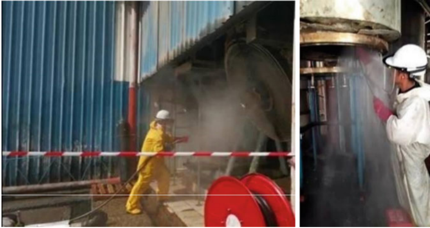
Fig. 20 High pressure jet cleaning of spiral heat exchangers
