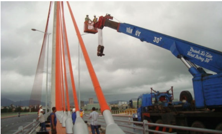
Fig. 3 Installation of the accelerometers for damping test on the Tran Thi Ly stay cable bridge (photo provided by VSL Vietnam)
