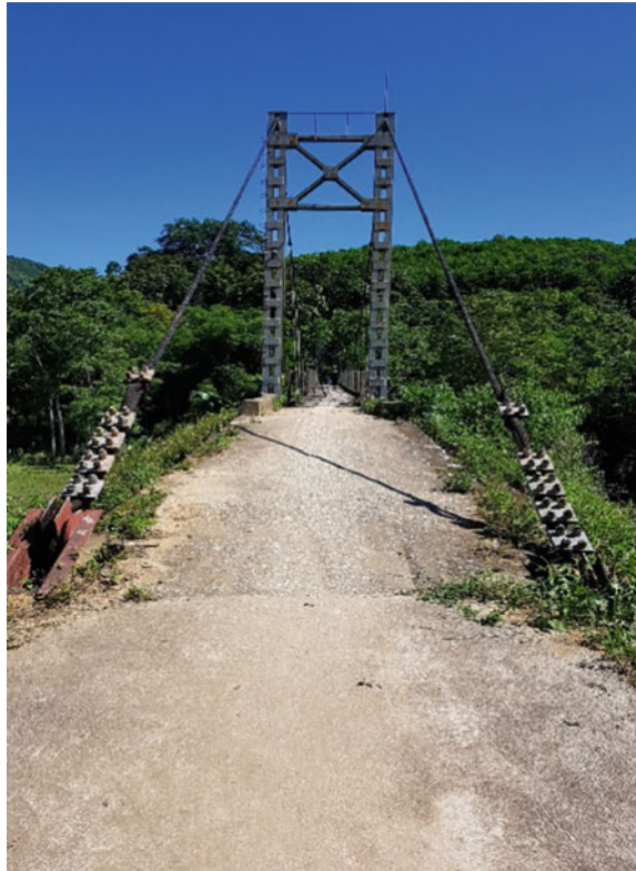
Fig. 2 Overall view of the bridge
