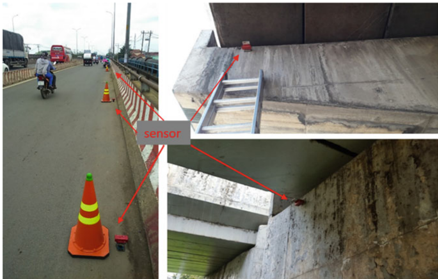
Fig. 5 Data collection (deck, pier, and abutment)
