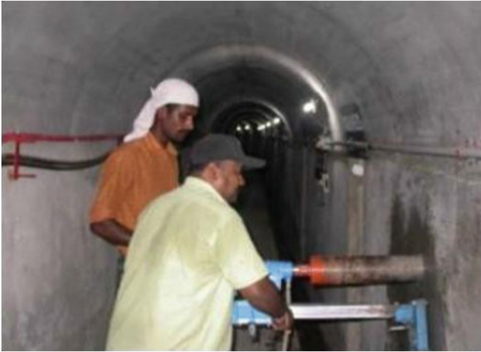
Fig. 3 Core extraction process from concrete dam [13]
