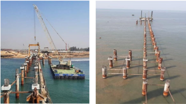
Fig. 2 Barge and Jack-up barge positioning and alignment of piles
