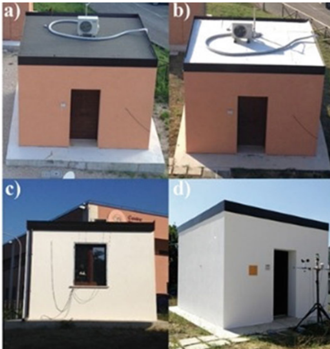
Fig. 1 Original prototype building (a) and implementation of a cool membrane (b) and cool painting (c, d) [61]
