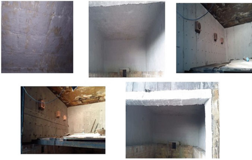
Fig. 2.8 Furnace after installation of pyro block
