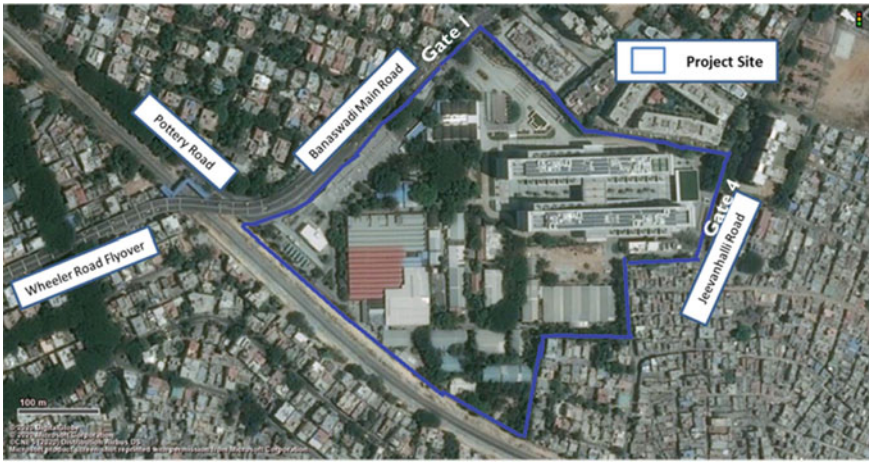
Fig. 1 Project site and the adjoining roads
