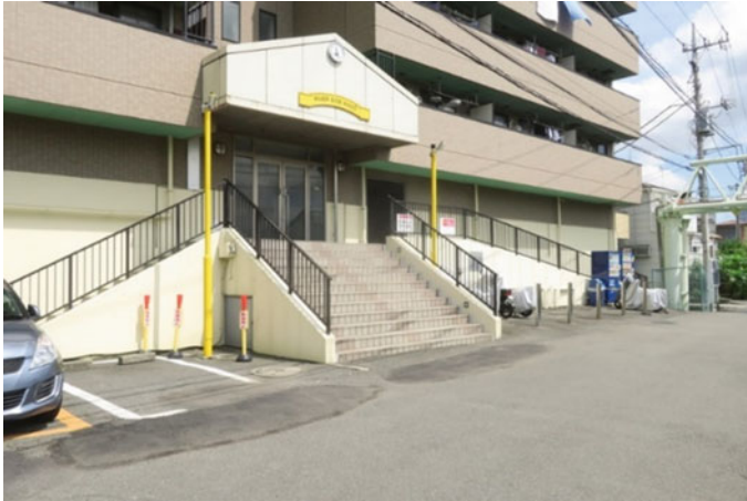
Fig. 4.55 Apartment building resting on elevated foundation
