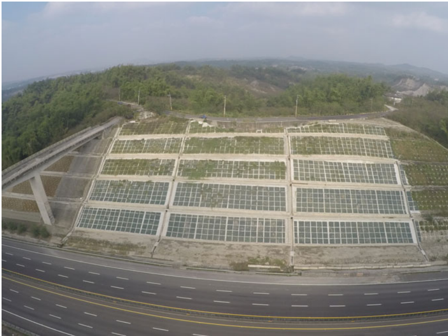
Fig. 7.9 Slope after repairing
