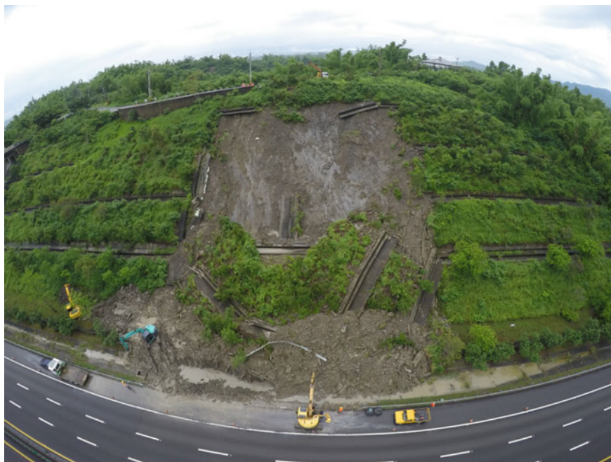
Fig. 7.6 Failed slope
