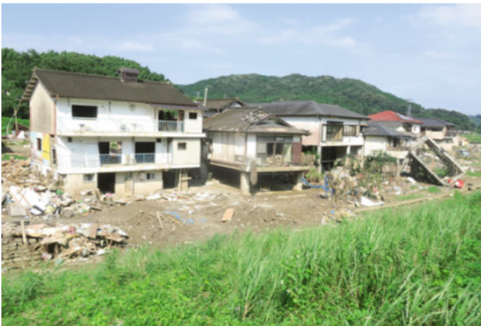
Fig. 4.49 Houses in Kuma Village near Hitoyoshi City damaged by the flood disaster in July 2020
