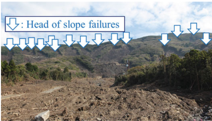
Fig. 4.2 Rainfall-induced slope failure in Izu Oshima Island, Japan, in 2013
