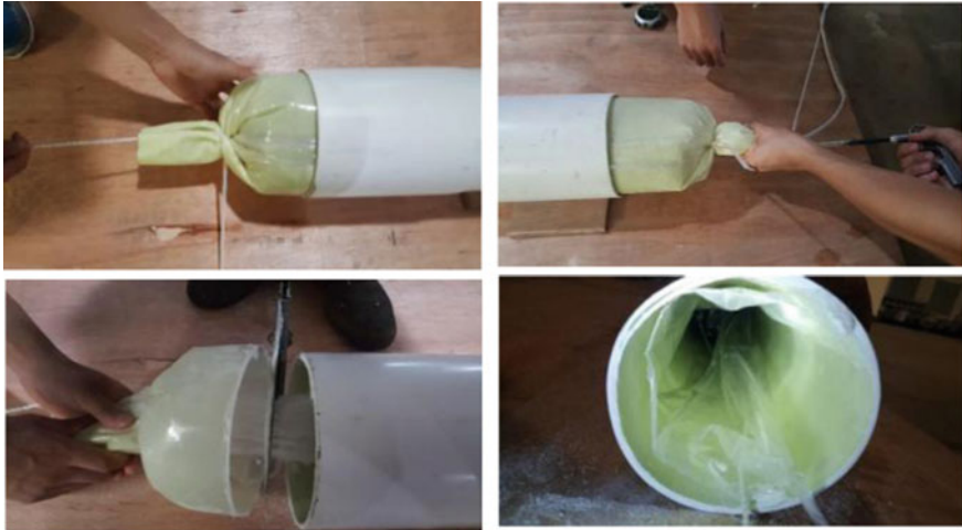
Fig. 3 Lining repair of small diameter pipeline
