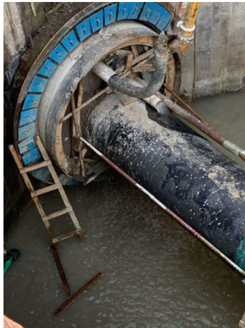
Fig. 2 Cement mortar injection into casing on site
