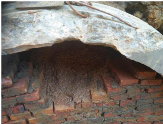
Fig. 3 On-site sand blowing
