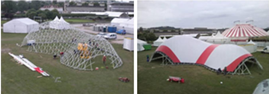
Fig. 2 Grid shell in composite materials for Solidays festival in Paris [2]
