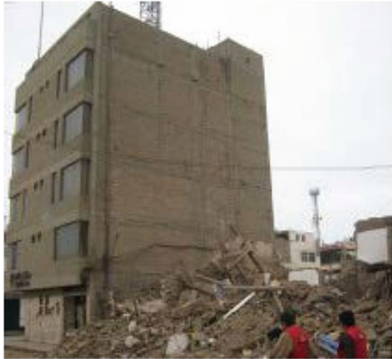
Fig. 6 CM building during 2007 Pisco, Peru earthquake [21]
