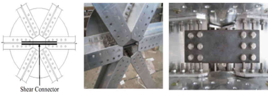
Fig. 6 Circular plated joint with shear connector [1]
