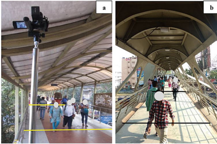
Fig. 2 a Skywalk facility and b FOB facility
