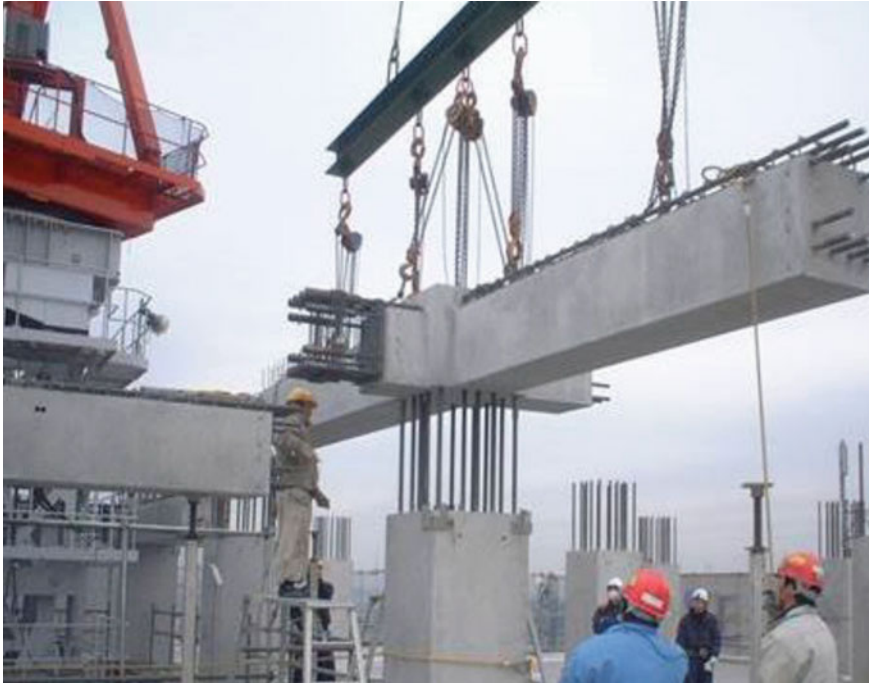
Fig. 1 Installation of lotus root precast beam–column connection [1]
