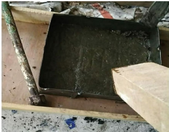
Fig. 4 Paver block placing and compaction in mould
