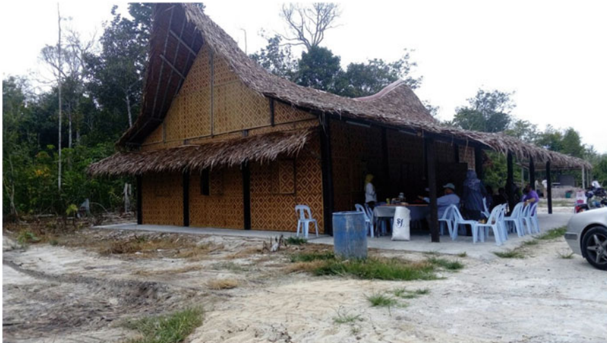
Fig. 10.25 The completed building photo
