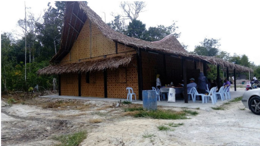
Fig. 10.25 The completed building photo
