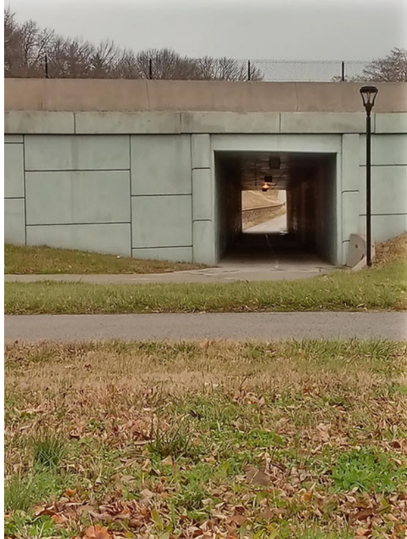
Fig. 9.1 An underground corridor at Saint Louis, MO that allows animals to migrate across a highway to other parts of the forest
