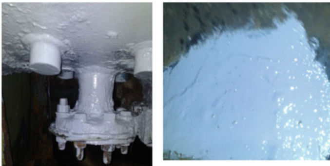
Fig. 6 After CorroKote application on cooling water pipe
