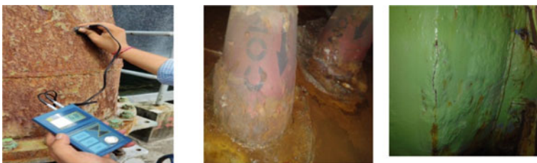
Fig. 4 Pipe thickness measurement
