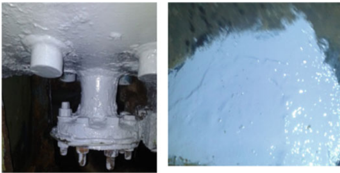
Fig. 6 After CorroKote application on cooling water pipe
