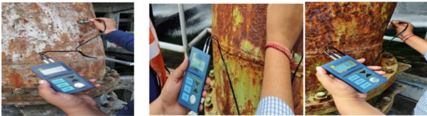
Fig. 3 Pipe thickness measurement
