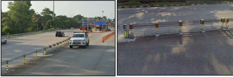
Fig. 1. Current moveable fence at exit toll Ayer Keroh, Melaka.
