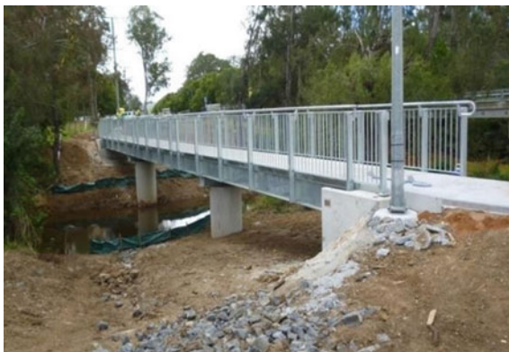
Fig. 27 Picture of pedestrian bridge casted in the rural area
