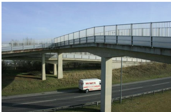
Fig. 25 Picture of foot bridge casted over the road
