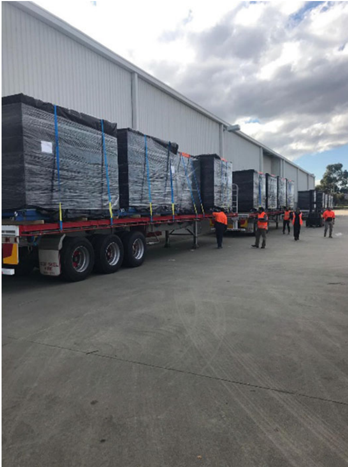
Fig. 3 Bathroom pods ready to be transported to site
