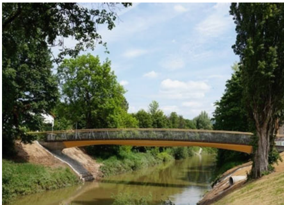
Fig. 26 Picture of foot bridge casted over the small canal
