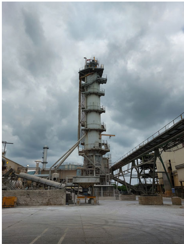
Fig. 42.8 A multiple shaft mixed-feed kiln and slaker
