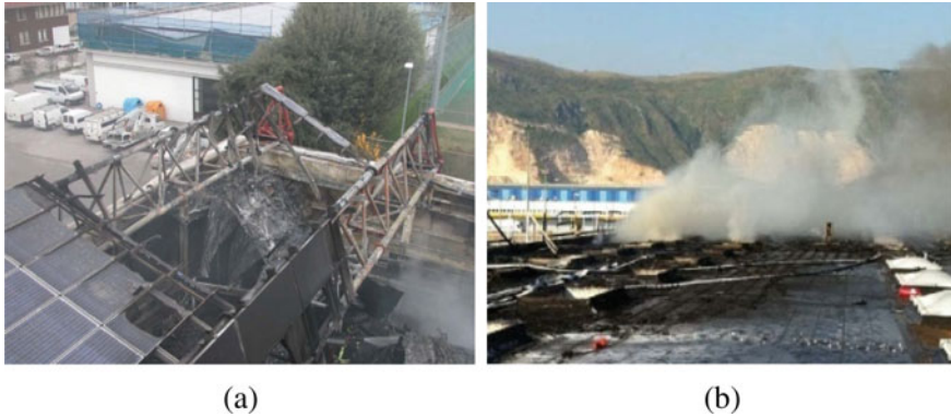
Fig. 7 a 1000m 2 warehouse fire and b externally ignited fire and propagated with the aid of installed PV system [15]
