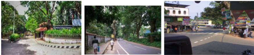
Fig. 90 Existing condition of Kattangal junction and nearby surroundings. Source Author
