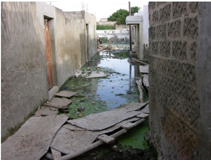
Fig. 3 Flooded houses in Pikine, Sénégal
