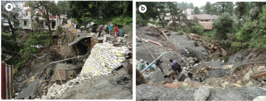
Fig. 15.8 a The crown portion of the landslide located on the Sher-ka-Danda hill slope damaging the narrow link road connecting Birla Vidya Mandir School with the town Mall Road; b downslope view of the landslide exhibiting the threat to the habitations
