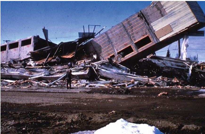
Fig. 4.7 Anchorage Westward hotel damaged by pounding in the Alaska earthquake of 1964 [9]
