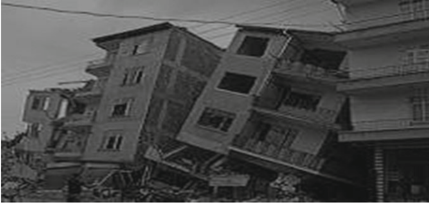
Fig. 4.8 Pounding damage in Caracas during the Venezuela earthquake of 1967 [8]
