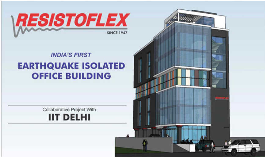
Fig. 1.42 Base-isolated showcase building (a collaborative project between Resistoflex and IIT Delhi)
