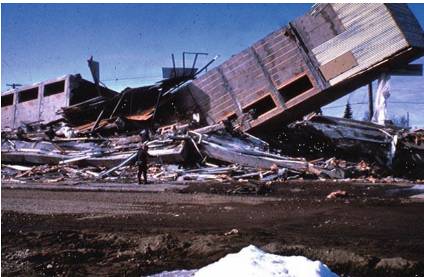
Fig. 4.7 Anchorage Westward hotel damaged by pounding in the Alaska earthquake of 1964 [9]
