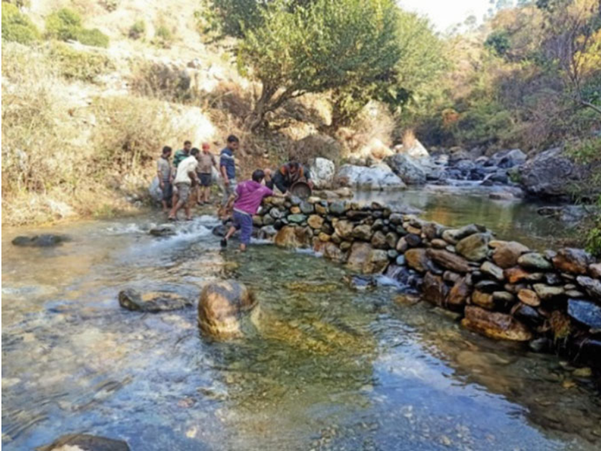
Fig. 10 Diversion weir and intake
