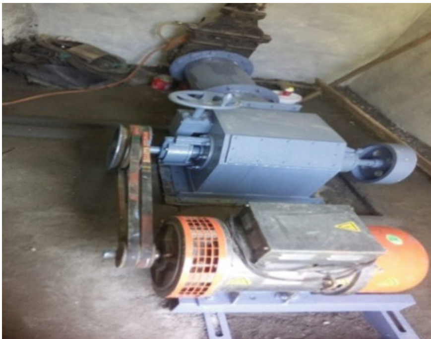
Fig. 14 Installation of turbine and generator
