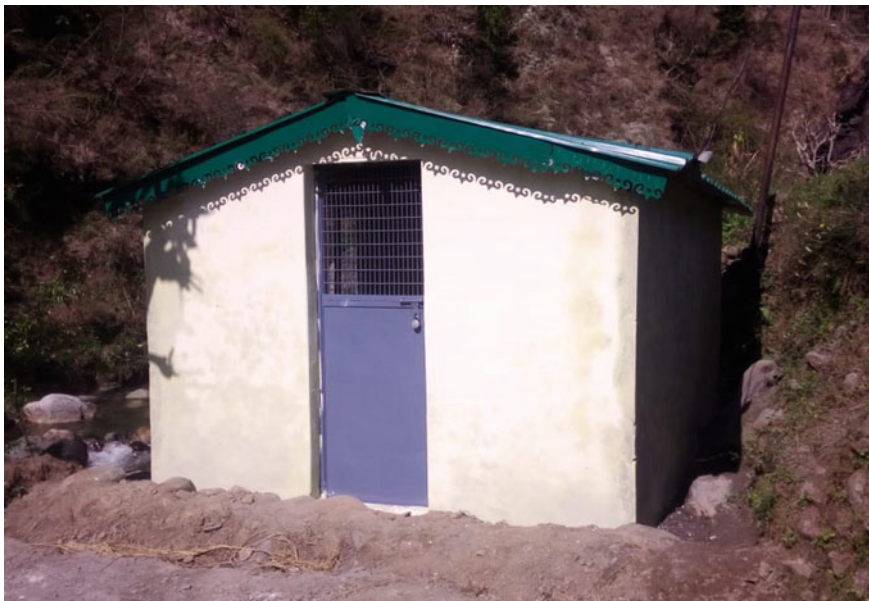
Fig. 13 Power house building
