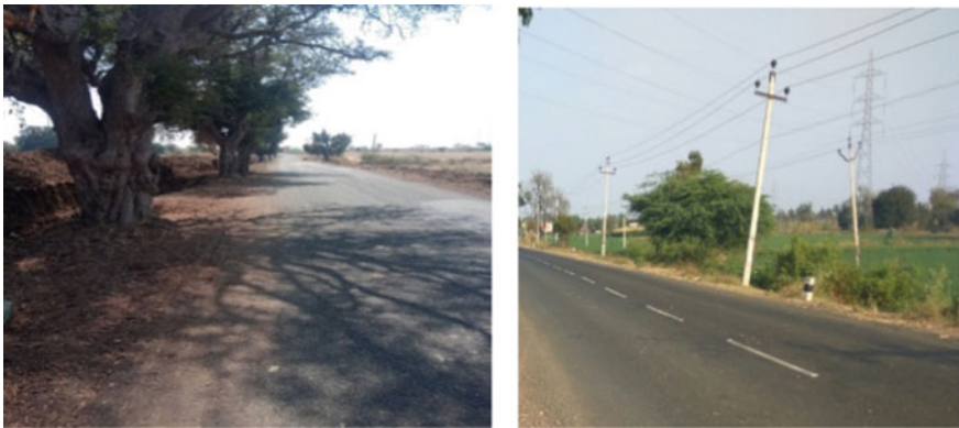
Fig. 3 Presence of trees and electrical poles along the roads
