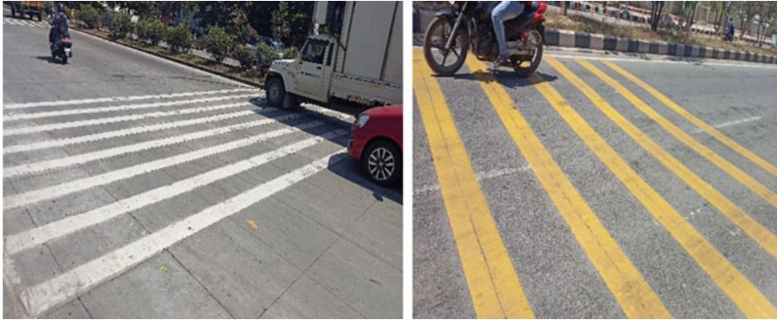
Fig. 2 Rumble strips and transverse markings
