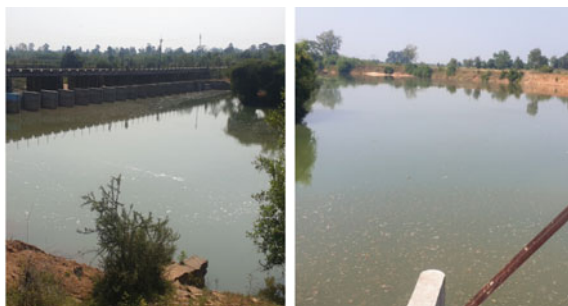
Fig. 22 BCB at Major Bridge Andhari Irrigation for 1600 acre by filling existing lakes for 16 lakh cub m using solar panels, cost 20,000 Rs per acre
