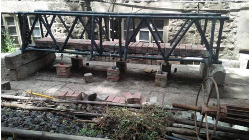
Fig. 1 04m bridge laid out for testing at CoE, Pune. The location of the deflection sensors can also be seen
