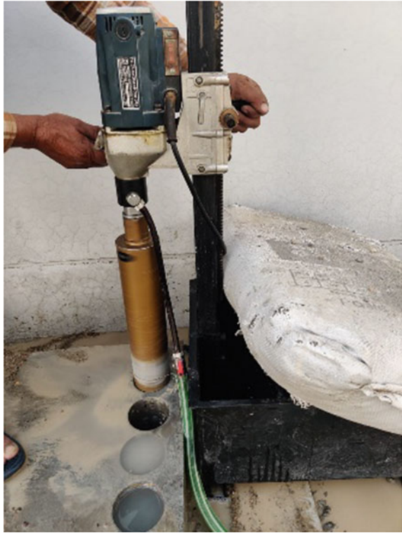
Fig. 8 Drilling cores from the slab
