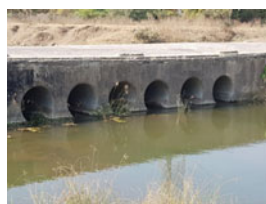
(a) A typical bridge1
