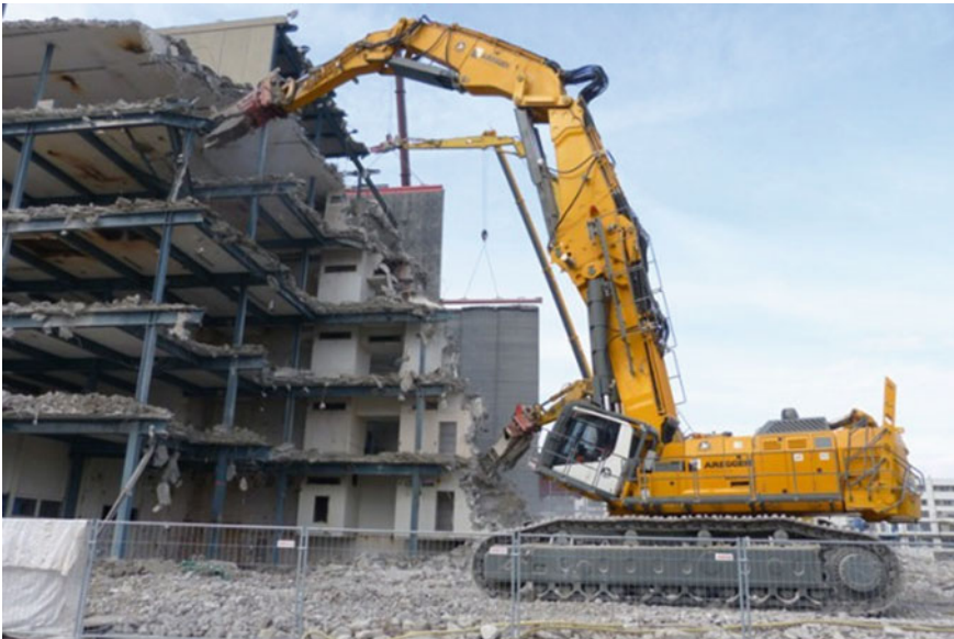
Fig. 1 Demolished concrete structures
