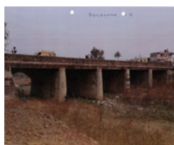
(b) A typical bridge2
