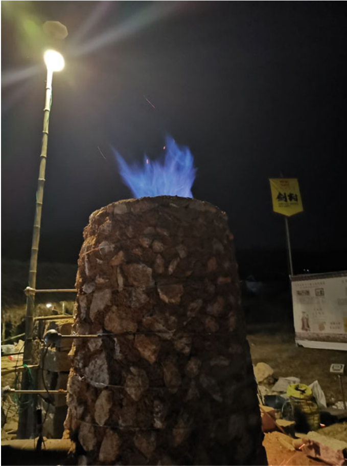
Fig. 7.11 Roast the furnace to dry off water in its interior
