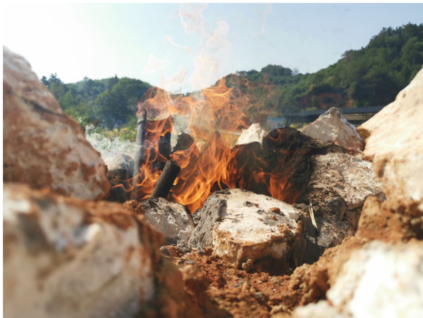
Fig. 7.9 Burn charcoal to roast the furnace to remove water content from the building material. It facilitates rapid temperature rise during iron smelting
