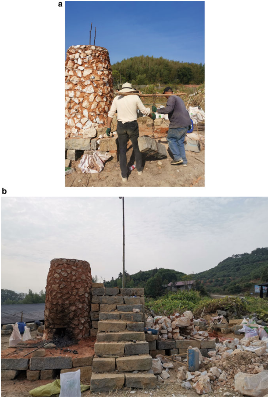
Fig. 7.10 Limestone footsteps were constructed for the convenience of ore feeding
