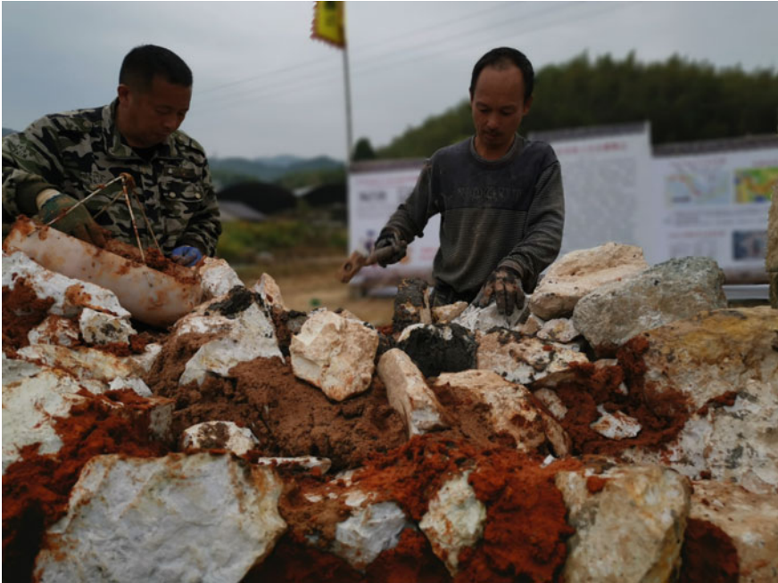
Fig. 7.8 Start building the furnace wall by piling up a mixture of fire clay and red clay with quartz
