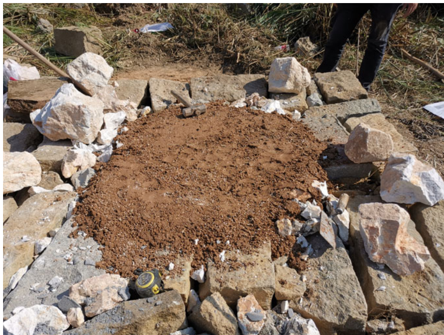
Fig. 7.7 The foundation of the furnace is crucial. The soil underneath the designated area for the furnace was tamped
