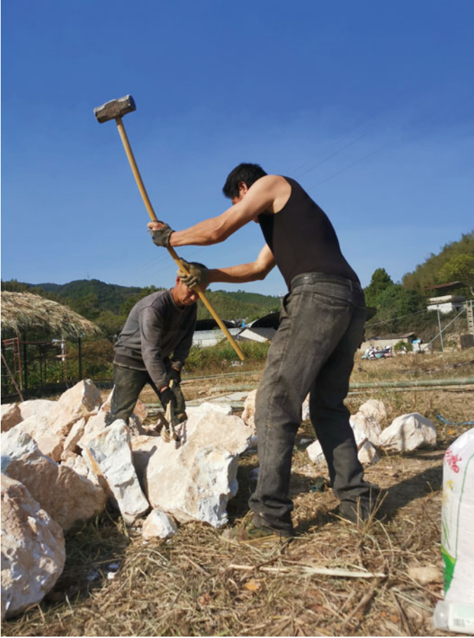
Fig. 7.6 Break quartz with a hammer to construct the furnace
