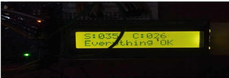
Fig. 4 LCD screen before leakage detection
