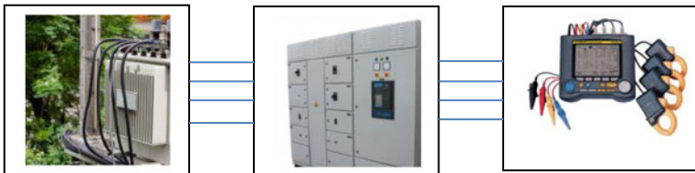
Transformer – 11 kV/415 V Power Distribution Board power quality analyzer
