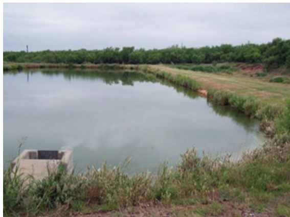
Fig. 2 Example figure for stabilization pond
