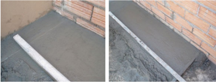
Fig. 5 Placing and compacting mortar with ruler
