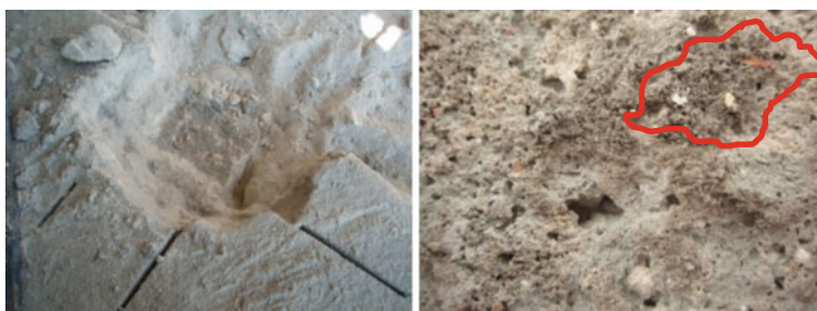
Fig. 10 Sample and concrete screed mortar contact plane
