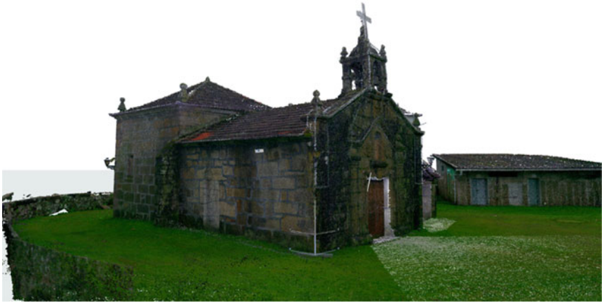
Fig. 2 Visualization of the imported global point cloud in the Teamwork Project (ArchiCAD Graphisoft)
