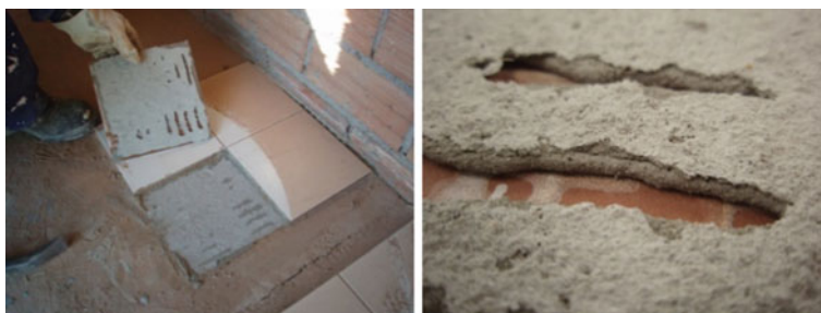
Fig. 9 Good adhesion of the adhesive to floor screed mortars
