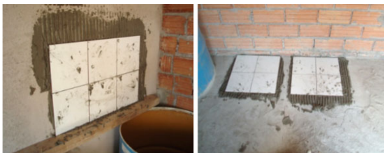
Fig. 6 Ceramic tile covering and flooring on both floors
