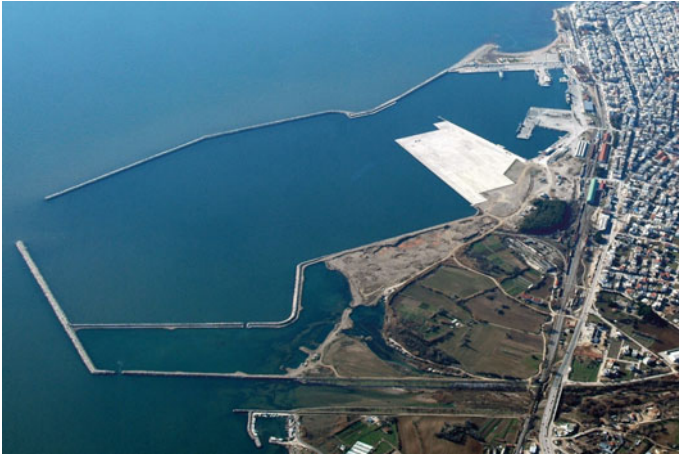
Fig. 2 Breakwater constructed at Alexandroupoli port, Greece [2]
