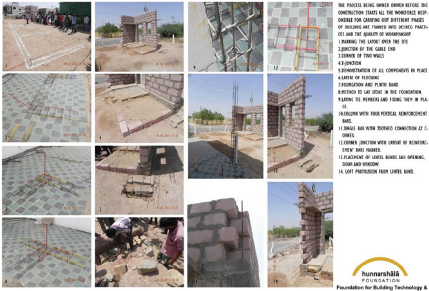
Fig. 4 Gujarati stone house details, Bhuj, Kutch (Documented by First Author)
