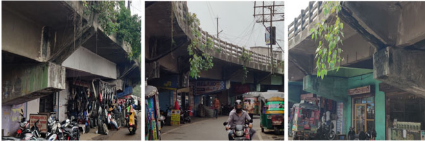
Fig. 1 Different reasons behind bridge fire events
