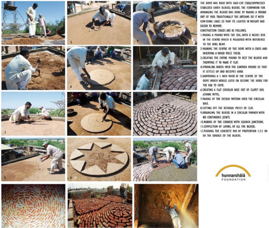
Fig. 6 Shallow brick dome construction process (Documented by First Author)
