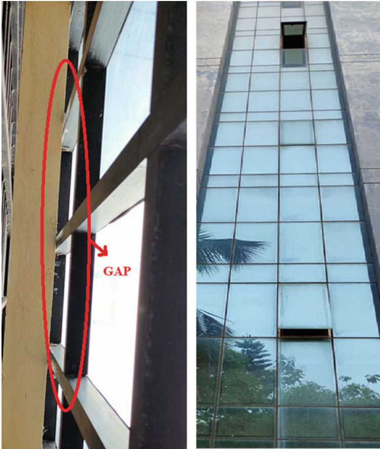
Fig. 12 Gap between slab edge and spandrel, and front elevation
