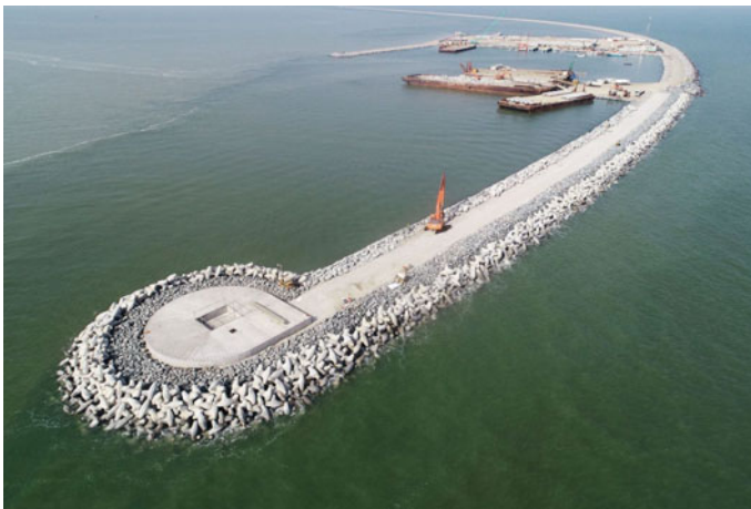
Fig. 1 Breakwater at Al-Faw grand port in Iraq-longest breakwater in the World [1]
