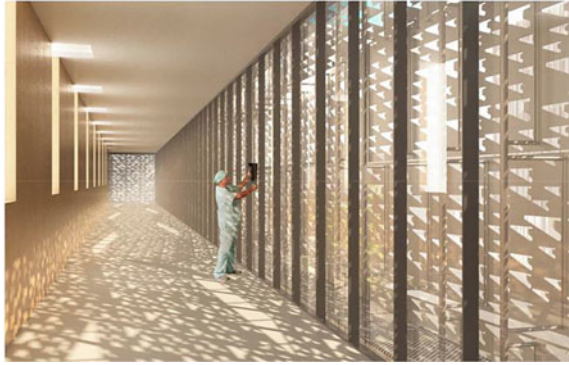
Fig. 5 Conceptual rendering of the façade of the University Hospital CHU Nantes, France featuring bands of thermo-bimetal into which incisions ‘free’ the memory shape to provide shading. © ArtBuild
