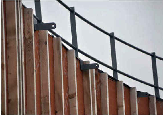
Fig. 17 Pho'liage fixing elements on the roof of the CIRC. © ArtBuild
