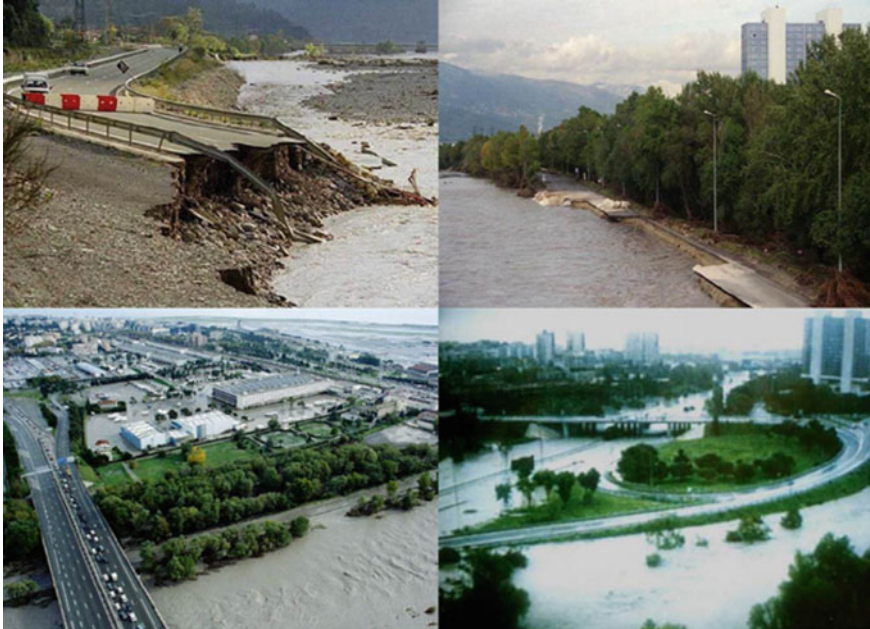
Fig. 79.2 Damages of 1994 flood event in Var low valley. Source Nice Matin [11]
