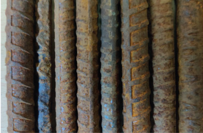
Fig. 3 TMT rods placed on conveyor belt view
