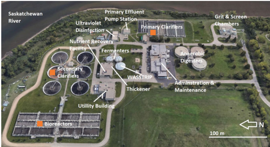
Fig. 1 Saskatoon Wastewater Treatment Plant (SWTP). WASSTRIP = Waste Activated Sludge Stripping to Recover Internal Phosphate. Bioreactors include anoxic, anaerobic and aerobic processes in different basins. The orange squares represent the approximate sampling locations used for experiments
