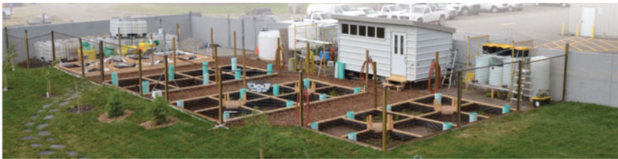
Fig. 1 Okotoks bioretention research site after construction and planting
