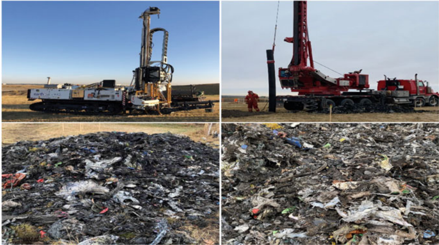
Fig. 1 Drilling rigs and excavated material
