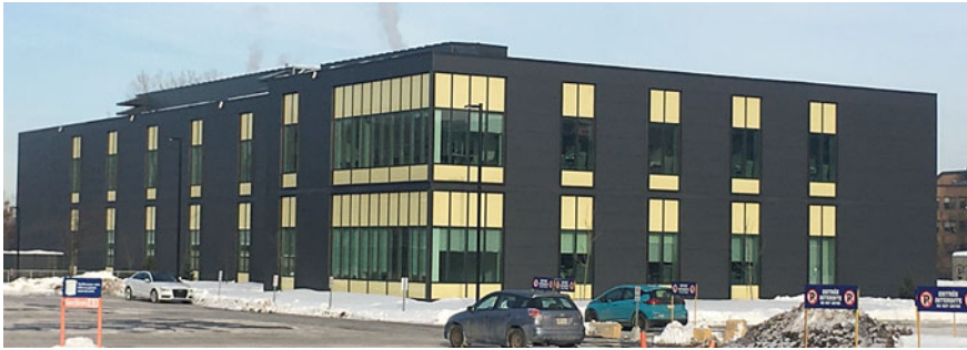
Fig. 1 The Maisonneuve-Rosemont Hospital expansion project
