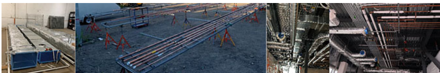
Fig. 3 Factory-assembled and on site installed MEP systems
