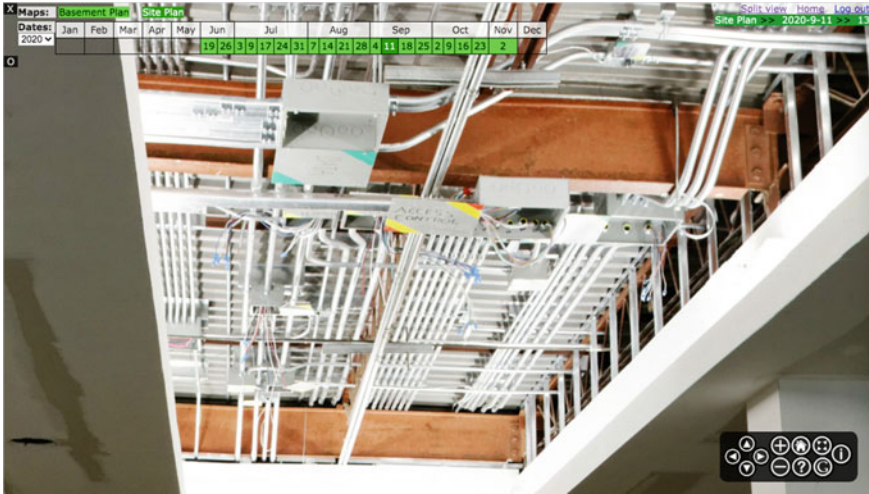
Fig. 3 Panorama location 13 ceiling detail
