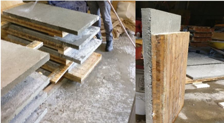
Fig. 2 CLT-Concrete composite sections after removing formworks
