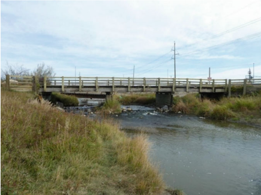
Fig. 1 The old Laycock Park Pedestrian Bridge
