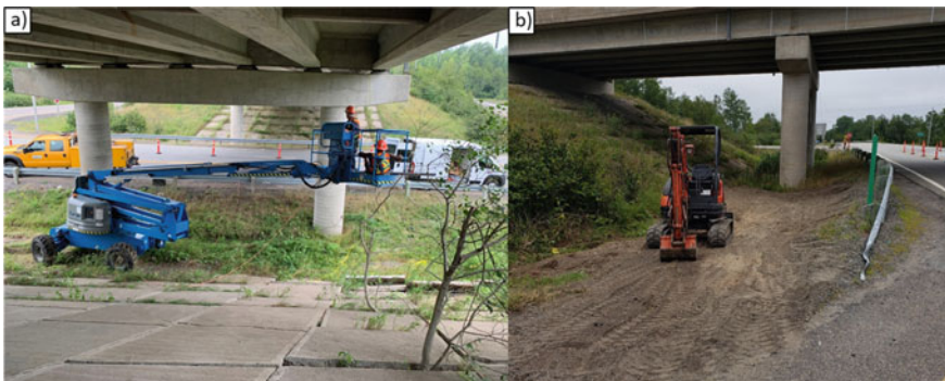
Fig. 3 a boom lift utilized for project. b temporary earth ramp
