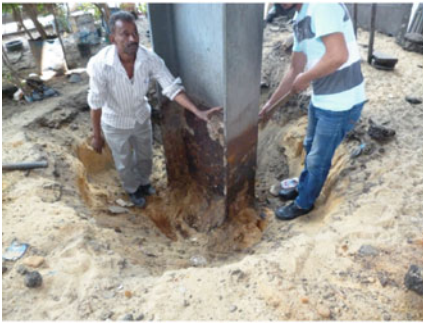
Fig. 11 Corrosion at bottom of bridge columns
