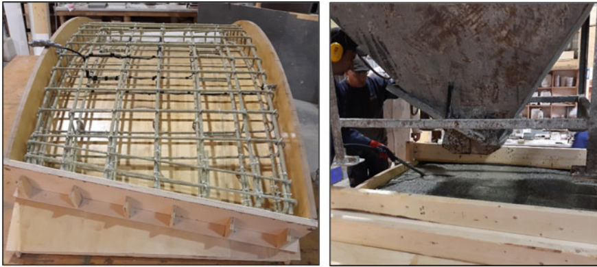
Fig. 2 Casting of the test specimens
