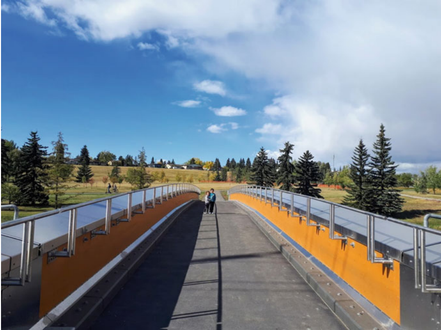
Fig. 11 Bridge aesthetic features including granite curbs and stainless-steel caps and bikeraill
