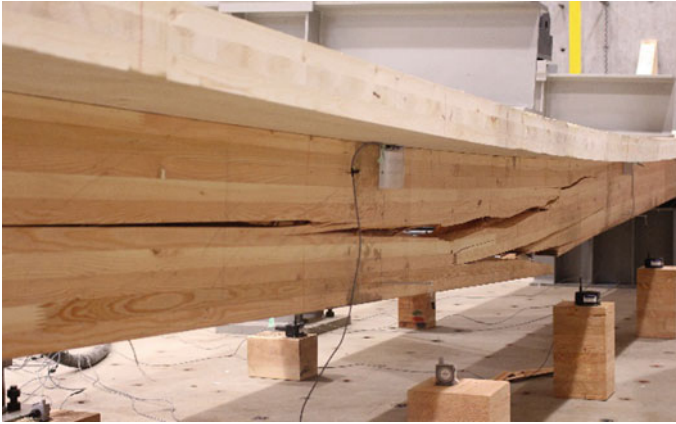
Fig. 6 Typical failure in Type A floor specimen
