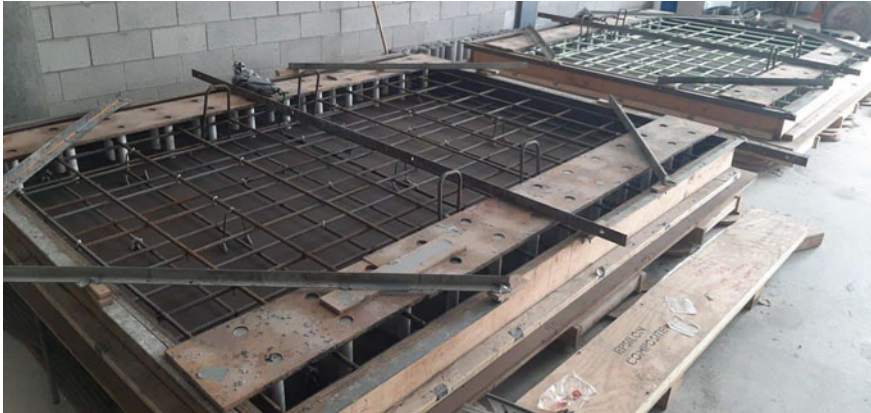
Fig. 2 Overview of the assembled GFRP meshes and formworks prepared for casting
