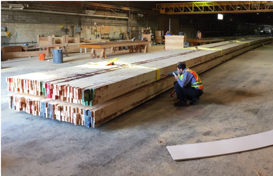
Fig. 5 Girders during fabrication
