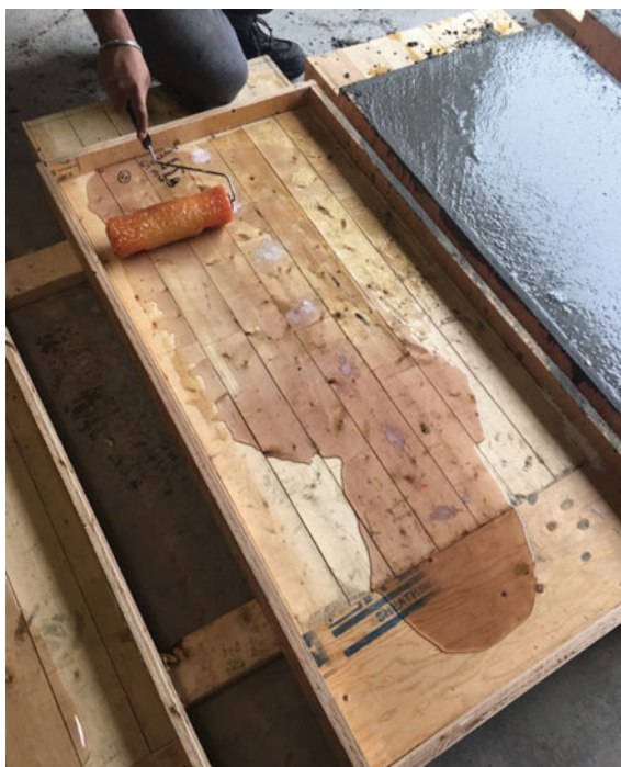
Fig. 1 A CLT panel with concrete formwork installed to allow concrete casting
