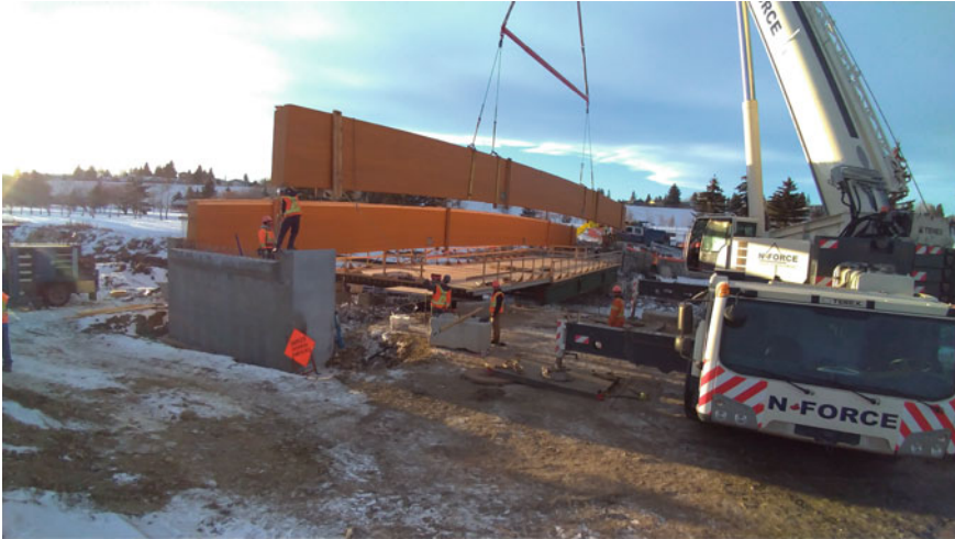
Fig. 6 Installation of glulam girders
