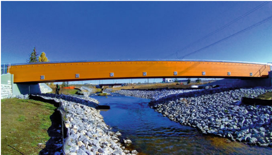
Fig. 4 Completed Laycock Park Pedestrian Bridge, looking North
