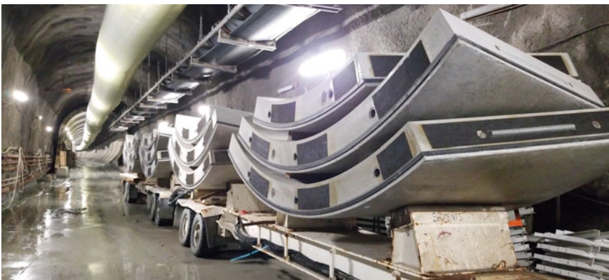
Fig. 10 RTV transporting PCTL to the tunnel heading
