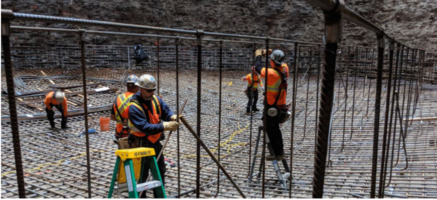
Fig. 5 Shaft 3 base slab reinforcement
