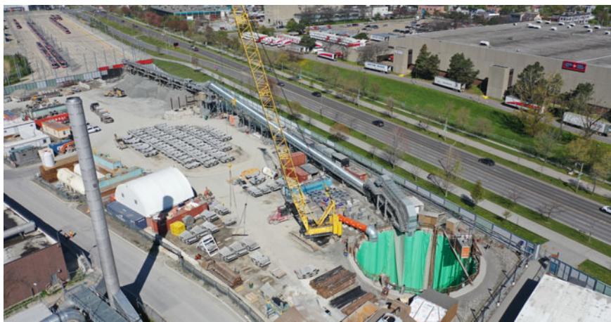
Fig. 12 Aerial of the vertical shaft conveyor and muck storage at Shaft 1
