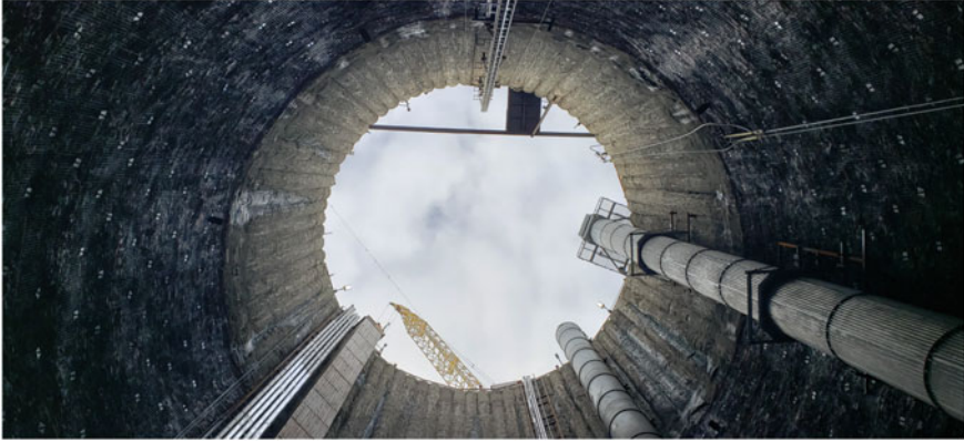
Fig. 4 Shaft 1 looking up showing secant piles and rock bolts
