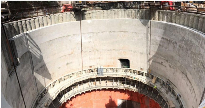
Fig. 6 Shaft 3 finished cast-in-place concrete and steel formwork supported by strand jacks
