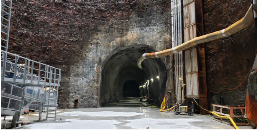
Fig. 7 Looking down the tail tunnel from within Shaft 1
