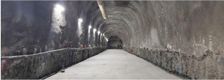
Fig. 8 Looking down the starter tunnel prior to TBM assembly
